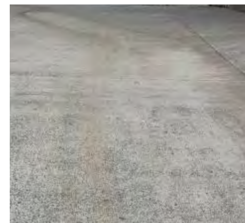
3 EXISTING YARD FINISH
